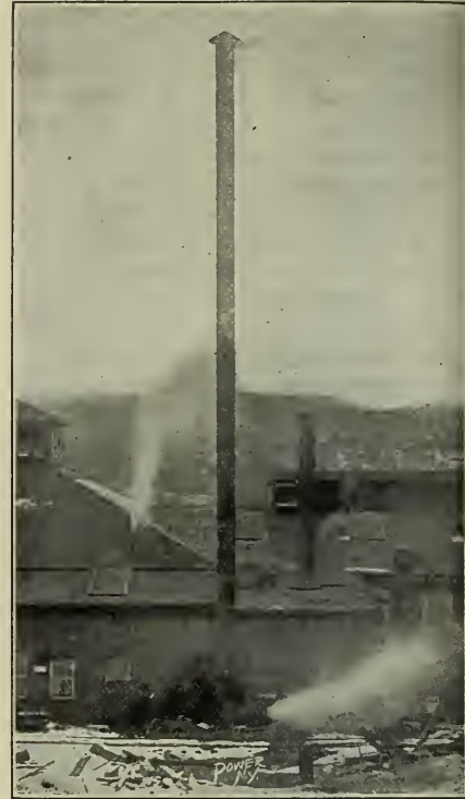
FIG. 4. THE OLD AND THE NEW STACK
